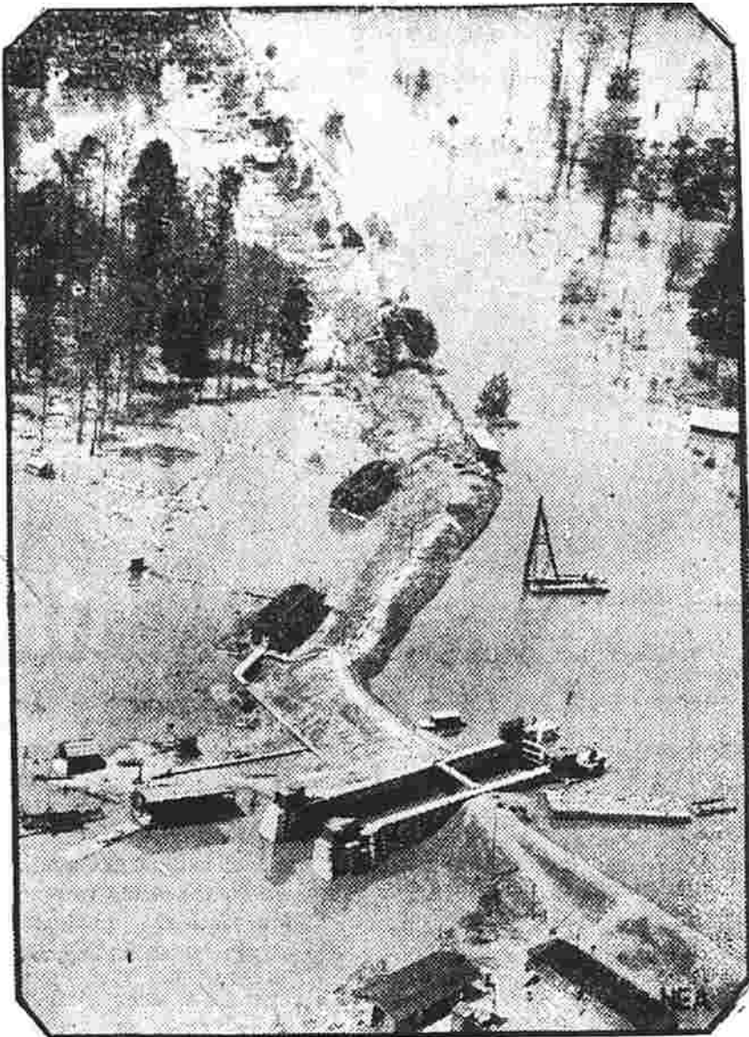
Airplane Photo, Copyright, 1927, NEA Service. The thin wall of earth shown in the remarkable airplane view above keeps two rivers, the St. Francis and the Little, and the thousands of acres of backwater from flowing down and inundating Marked Tree, Ark., where hundreds of refugees have concentrated. Recently a gun battle occurred at the lock when men from flooded towns tried to dynamite the levee and thus dry up their towns at the expense of Marked Tree.
